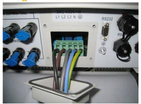
Cover the assembly, tightly screwed and then screw the cable gland
